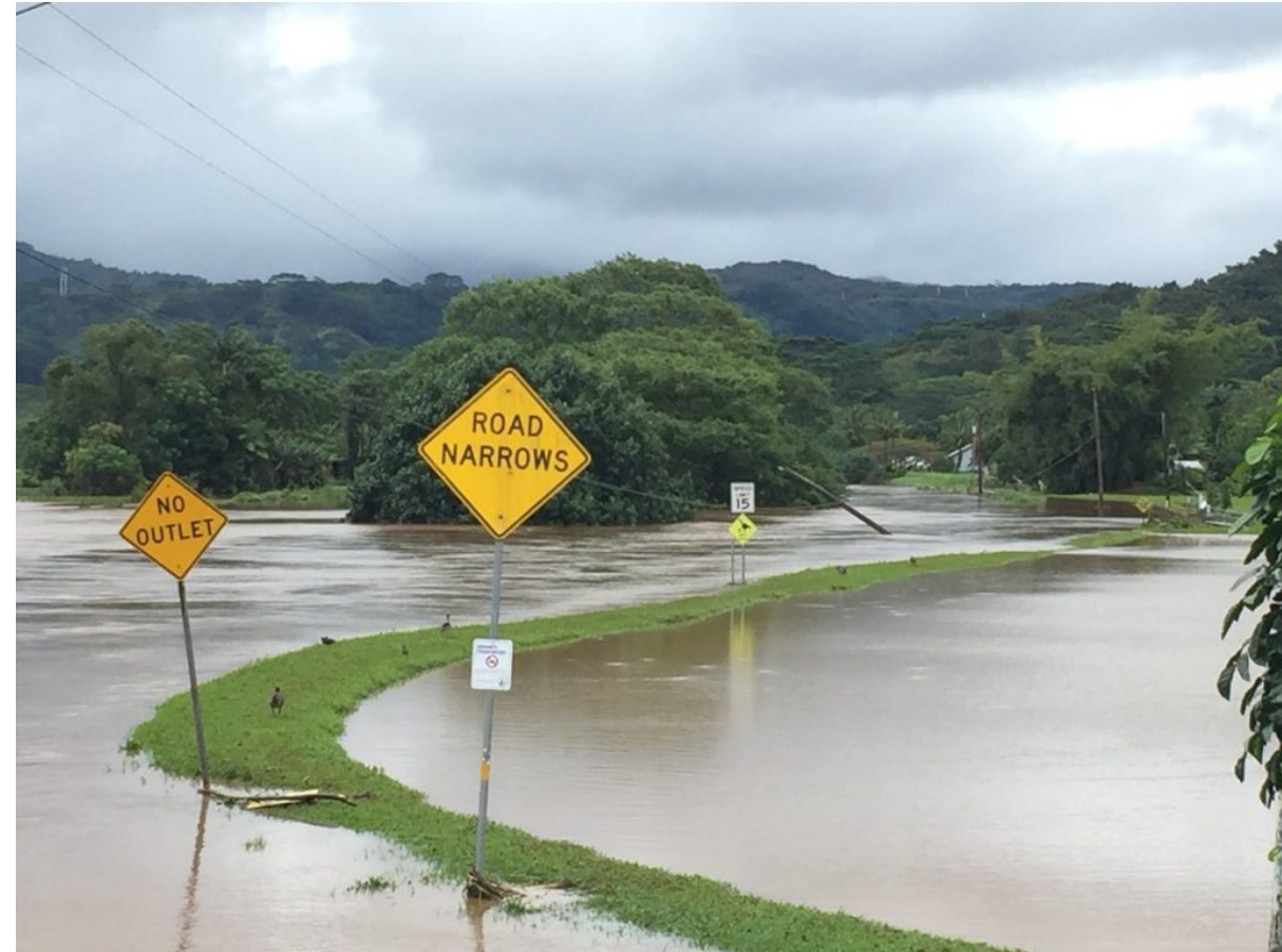
Flooded roads in Kaua'i , Hawaii, 15 April 2018. Photo: Hawaii DOT
