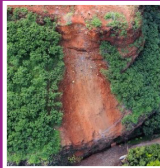
Roads and highways
