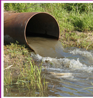
Water and wastewater systems
