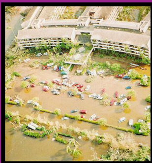
Over 8,000 people and 92 critical facilities exposed to Category 4 hurricane storm surge 5
